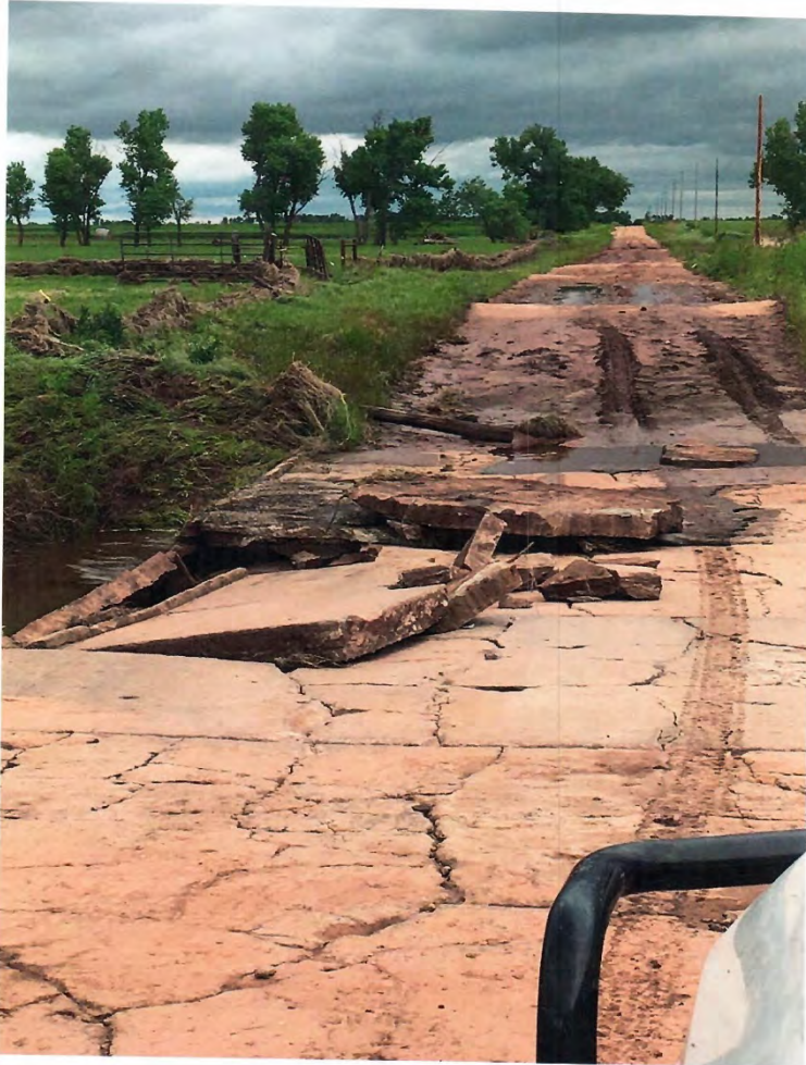
Concrete Failure Low Water Crossing
