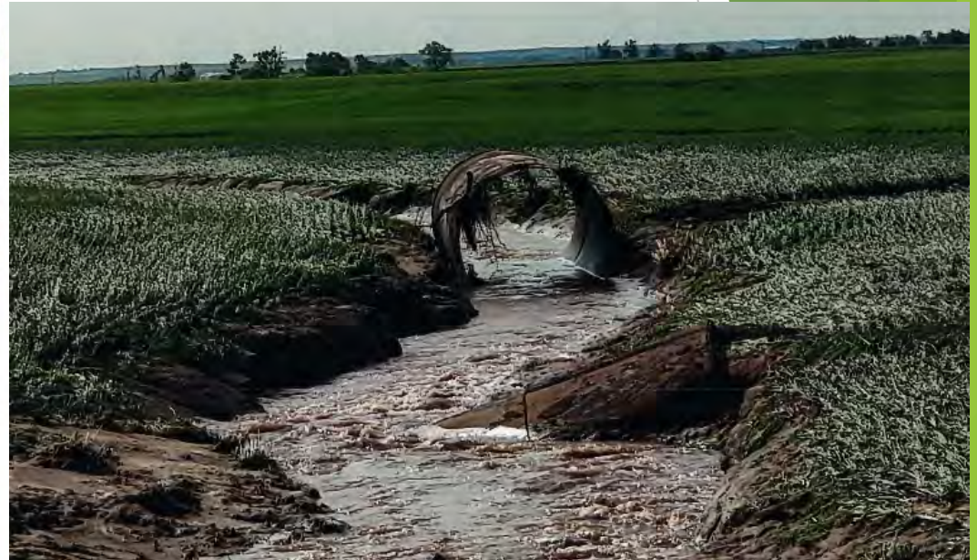
Cross Drain Pipe Washed Out Into Field
