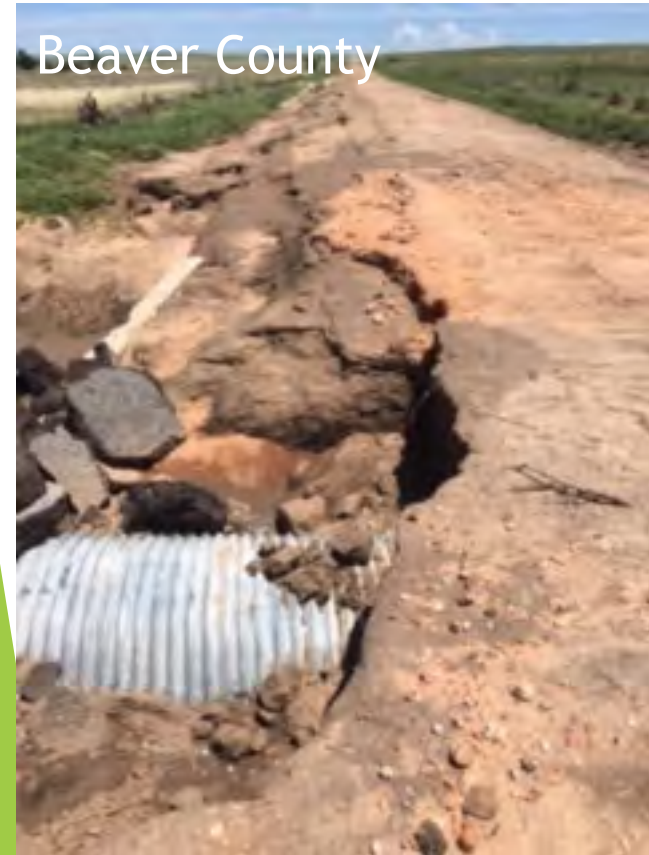
Erosion At Cross Drain Failure
