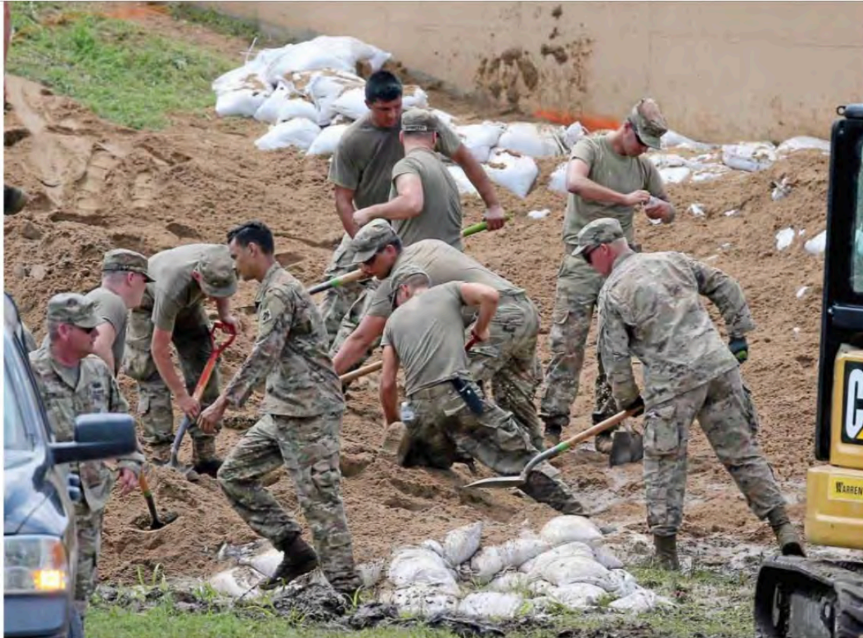
Service members with the National Guard and the Corps of Engineers work to fill sandbags behind a levee that was bubbling near West 67th Street and Charles Page Boulevard. TDM GILBERT/TUs a World
