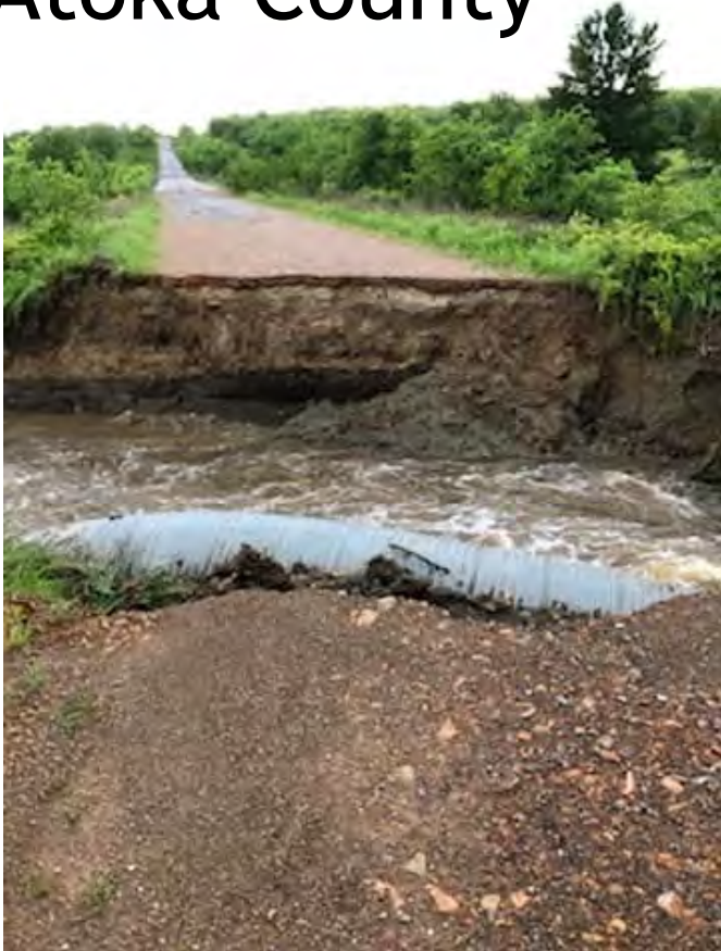
Cross Drain Failure
