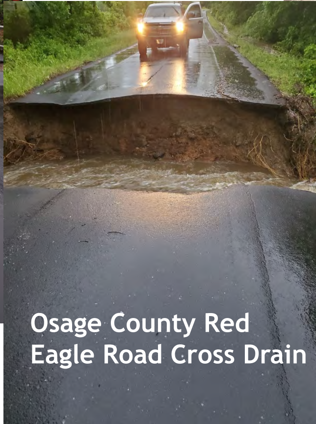
Osage County Peeling Asphalt off of Pavement
