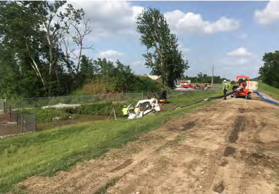
Army Corps pumps assisted to get water back into the river
