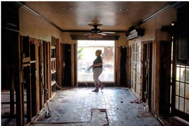
Teresa Tosh, director of county inspections, walks through the gutted living room of John Patterson's home in the Town and Country neighborhood west of Sand Springs during an inspection of the residence on Friday. JOSEPH RUSHMORE/for Tulsa World.
