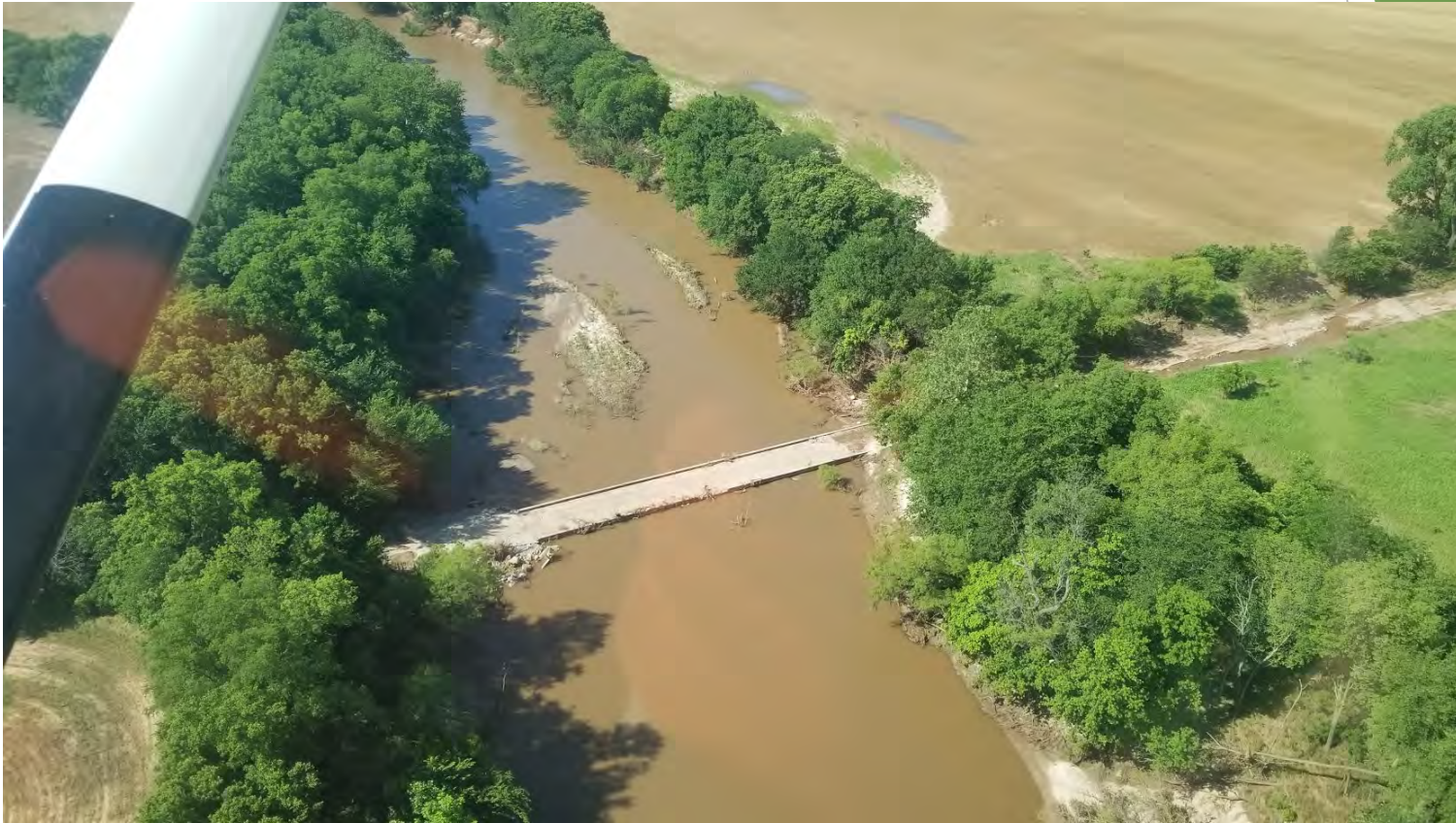
Grant County Bridge
