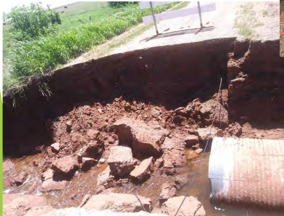
Harper County Cross Drain
